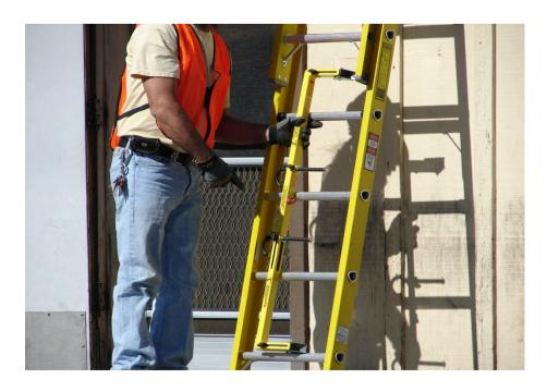
**6**. View bubble level to confirm whether ladder is set at proper 75.5 degree angle. Adjust ladder placement until bubble is at center of level window. (See picture below)
