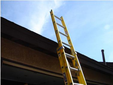
**3**. Setup ladder on as dry a surface as possible. If the surface is not level, it is recommended to use an approved ladder leveling device. (See picture below)
