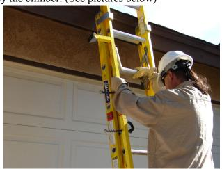
**8**. Clear debris, including loose gravel on rock roofs, leaves, or any other material that may prevent the feet from resting solidly on the roof surface. While on the ladder at roof level, carefully swing Safe T Climb device around horizontally against back of ladder and lower device down to roof surface. Both feet should be resting firmly on roof surface.
